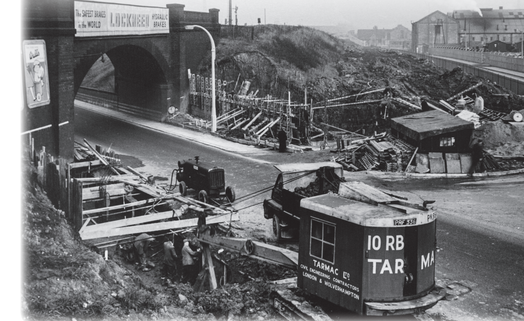
Excavation and foundations for the steel bridge over Liverpool Road – November 1956 – the Steelworks can be seen in the background
