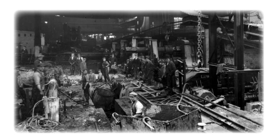
Construction began in 1911 and included buildings to house blast furnaces, coke ovens, steel furnaces, rolling mills, rod mills and offices. The canal infrastructure was important in the development of the new works. The MSC railway and building sidings were used to service the site, which had its own internal rail network to connect to the main line. A junction at the Irlam end was added in 1912 with further sidings following in 1913.
