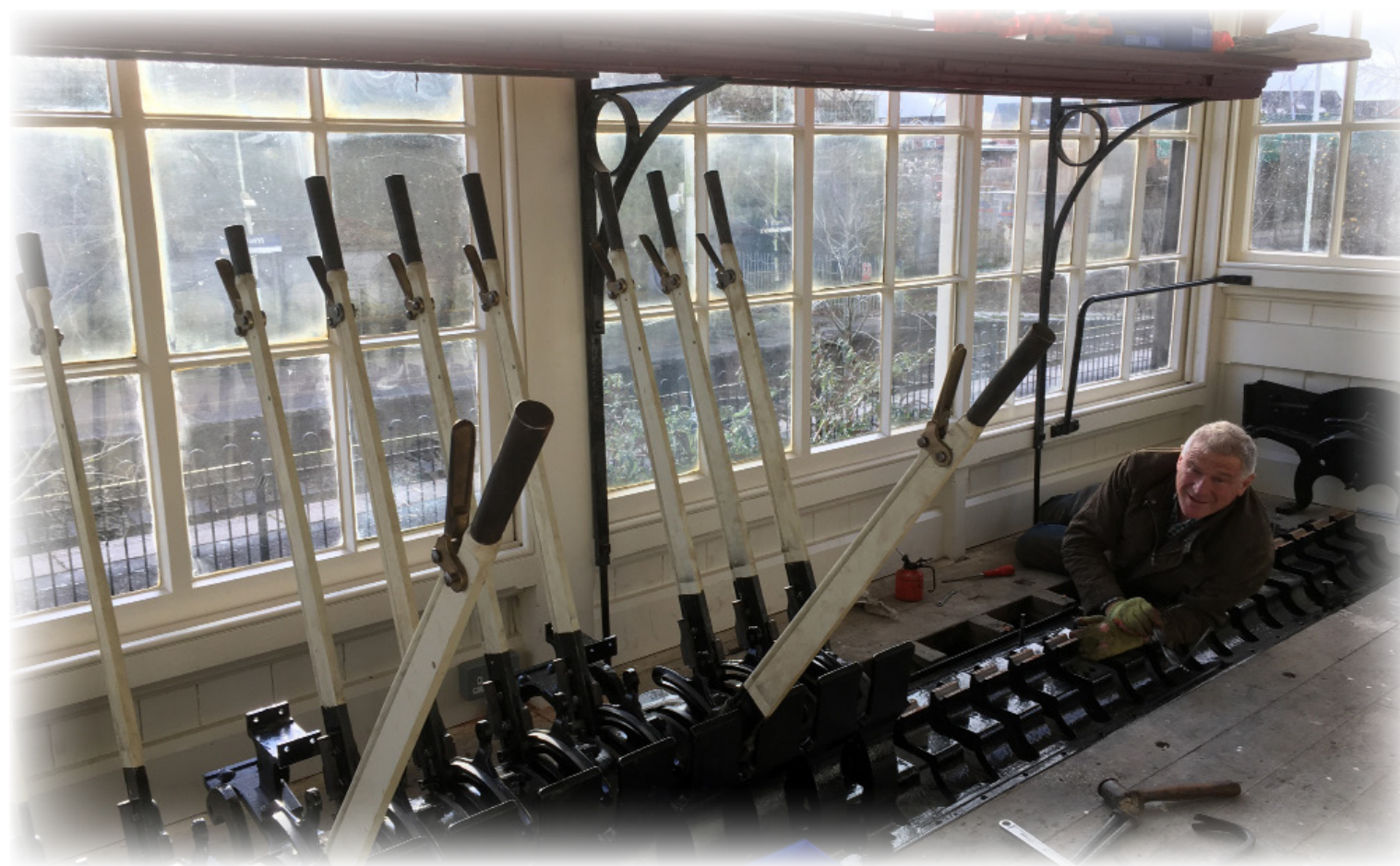
Neil McArthur installing the lever frame
