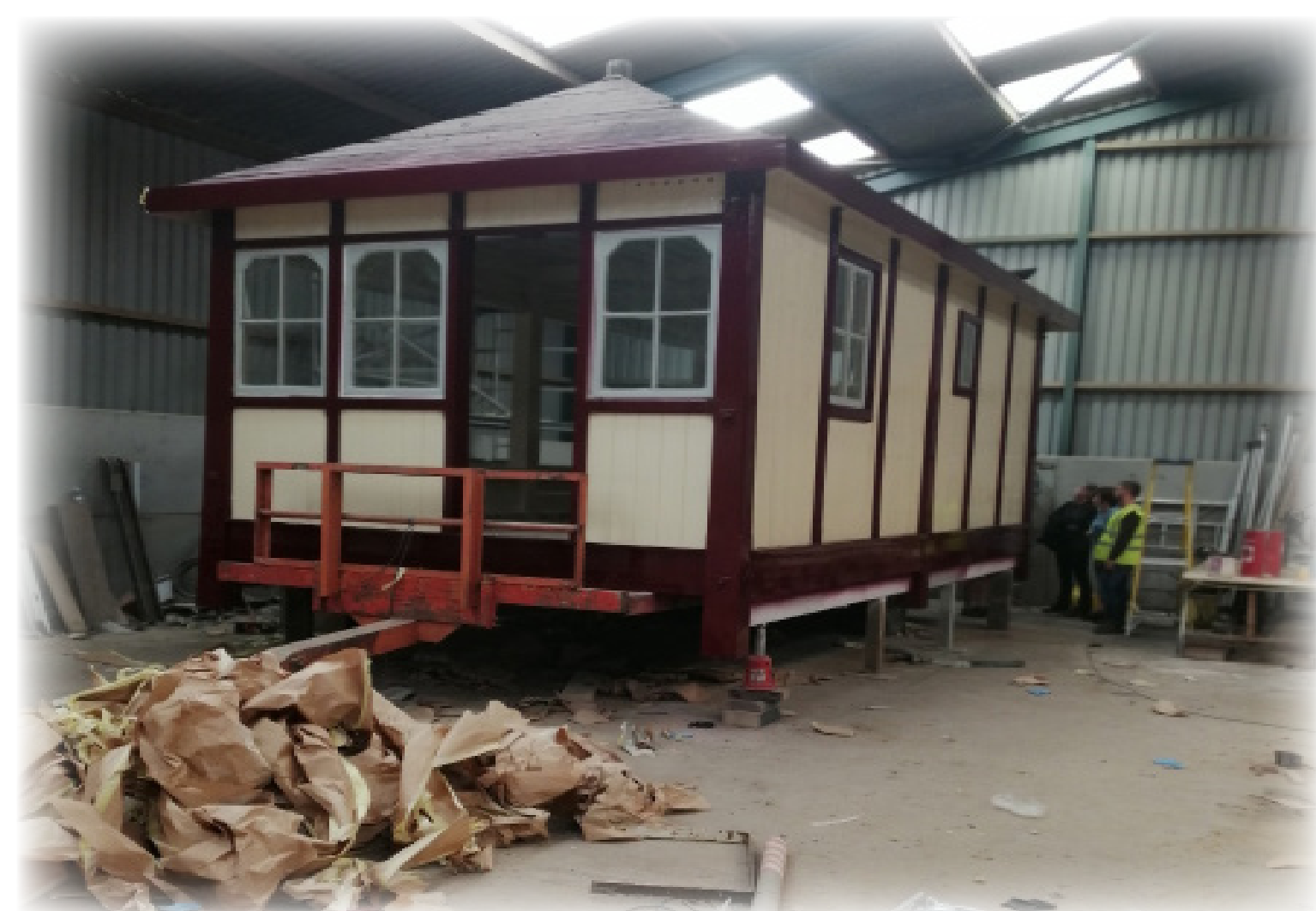
Upper floor of the Signal Box being repaired and restored
