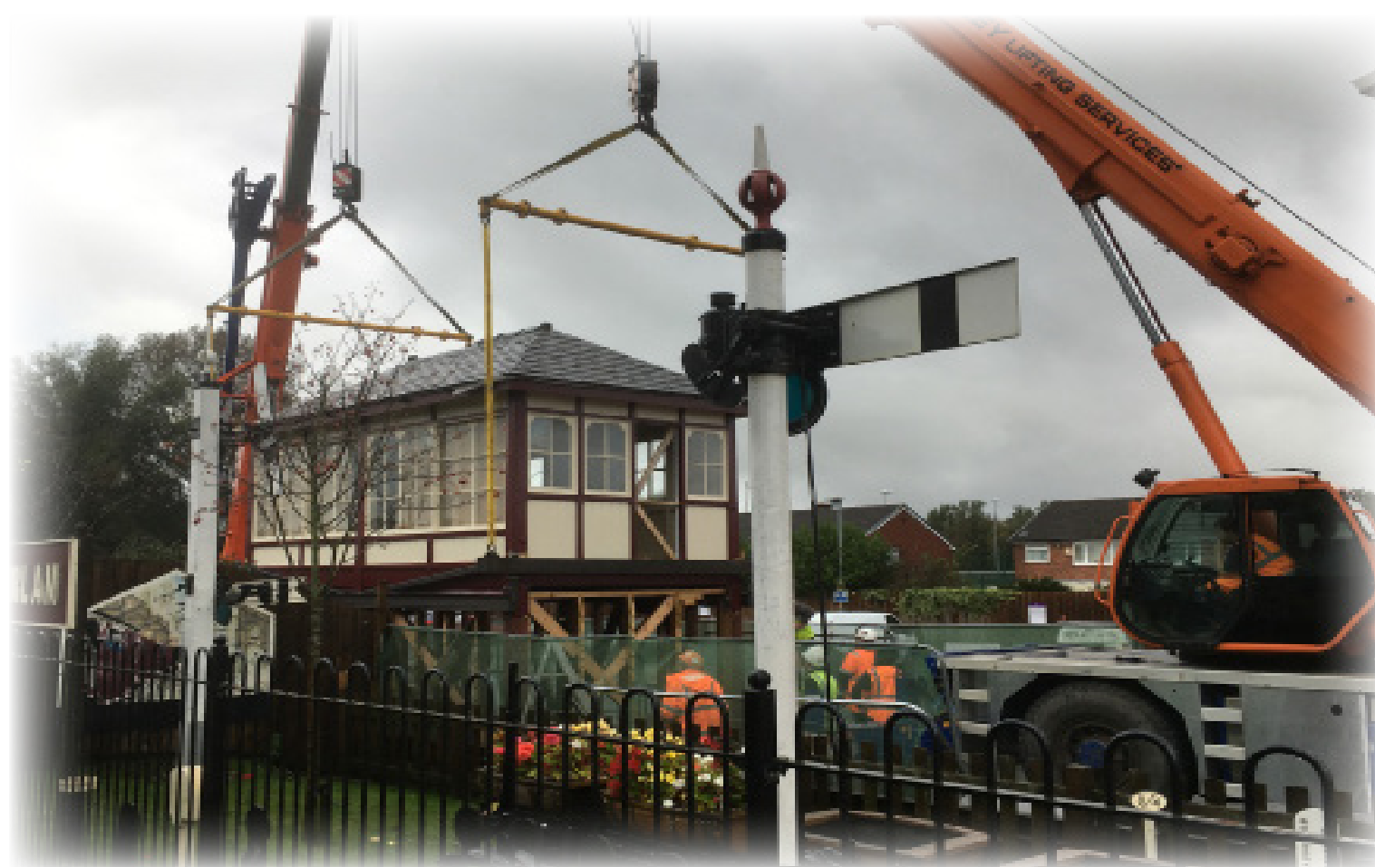
Signal Box upper floor being lowered and secured onto the lower floor re-construction at its new home at Irlam Station
