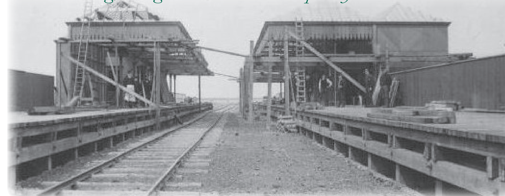
Cadishead's second station under construction in 1891. Both the buildings and platforms were of timber construction. The track seen running through the station is a temporary contractor's line.
